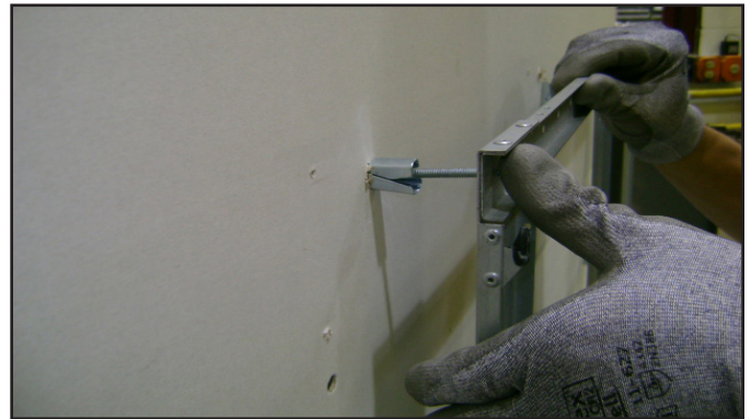
Figure 5 Installing Anchors in Hollow Wall
